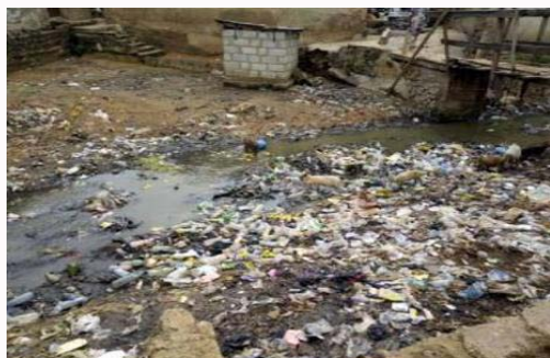
Figure 5: Showing Waste blocking Drainage and Stream Channels [41].
